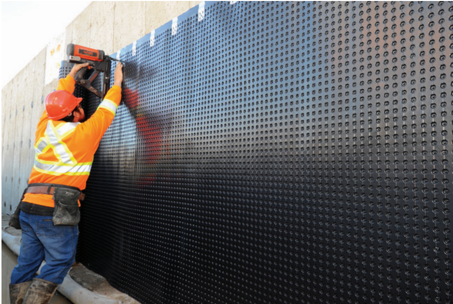
INSTALLING SPEEDCLIPS EVERY 30CM (12")
