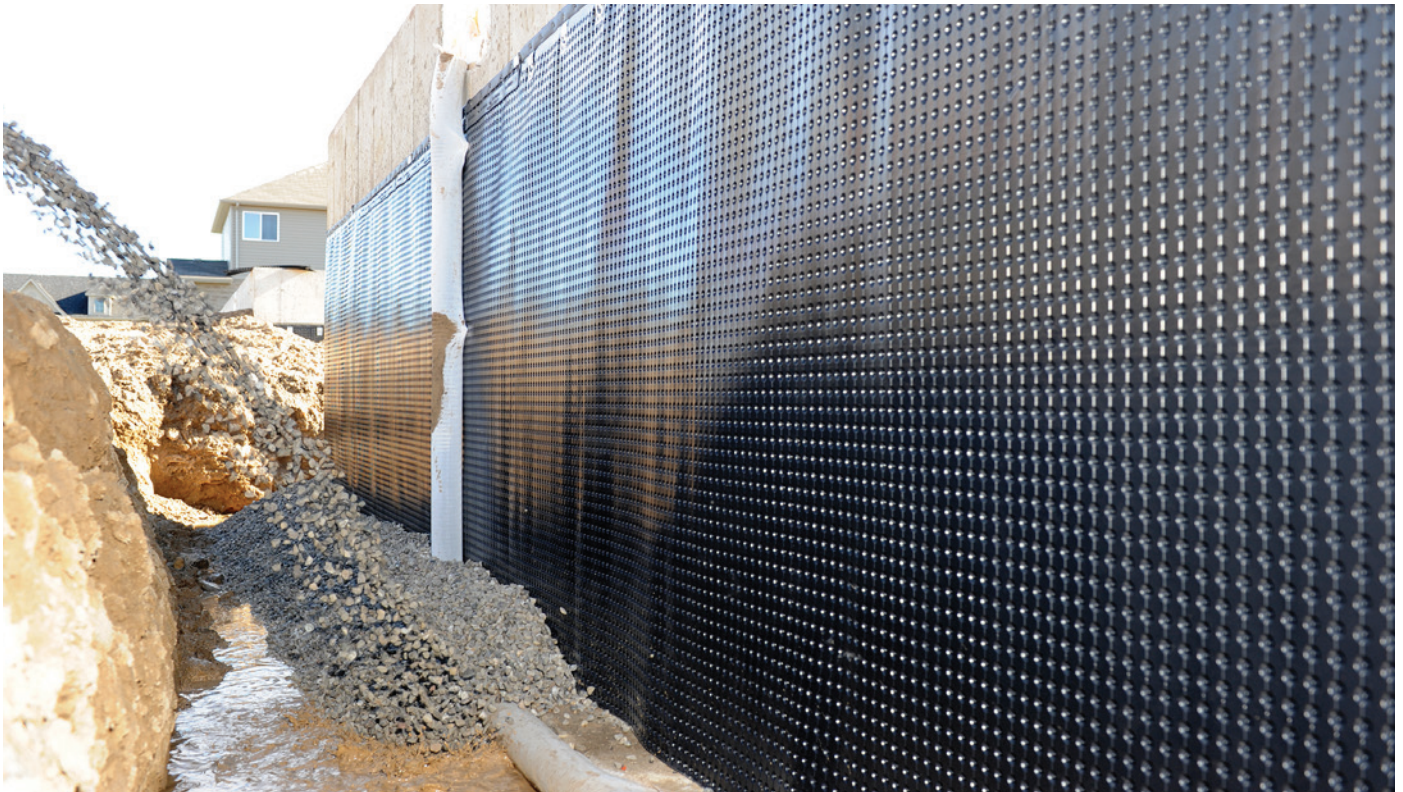
BACKFILLING OVER THE FOOTING DRAIN
