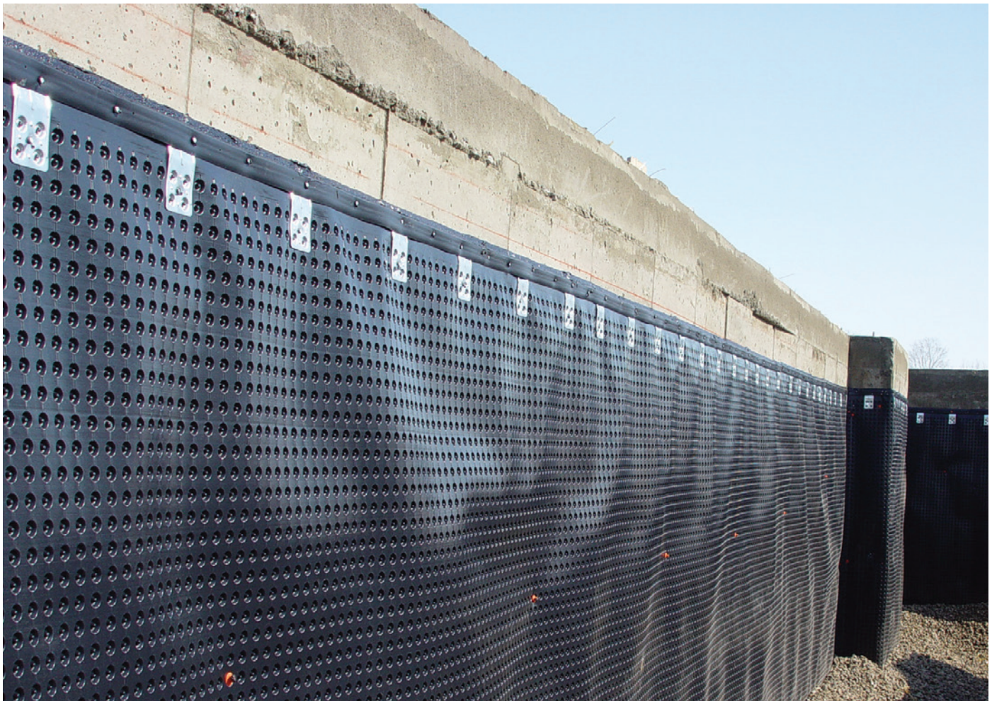
FINISHED INSTALLATION OF PLATON FOUNDATION WRAP
