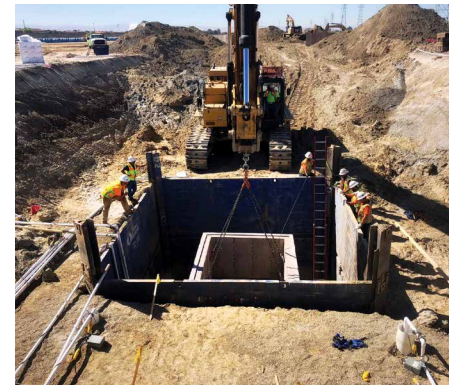
South Lathrop Commons, California, USA Wet Well/Pump Station • Xypex Bio-San C500, Xypex Megamix II with Bio-San
